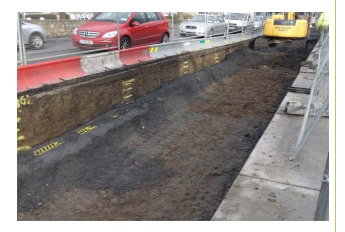
Project Details: Provision of a new quality bus corridor including full depth road construction & associated drainage & utility works incl footpaths
